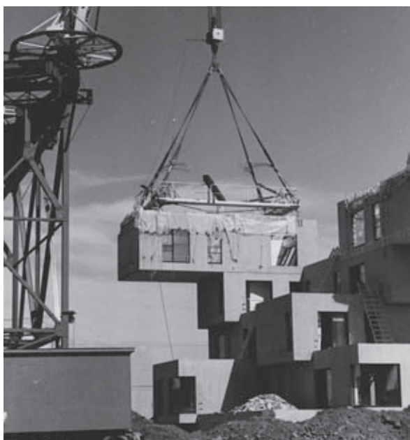
Habitat '67 majamoodulite paigaldamine kraanaga, Montréal, Québec, Kanada, 1966–1967. Safdie Architects
